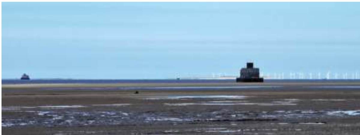
Figure 135: The two great Humber Mouth forts, Bull Sand Fort (left) and Haile Sand Fort (right), with Spurn Point in the background; begun in 1915, they were completed too late to be of much use in the First World War but were used in World War Two.
