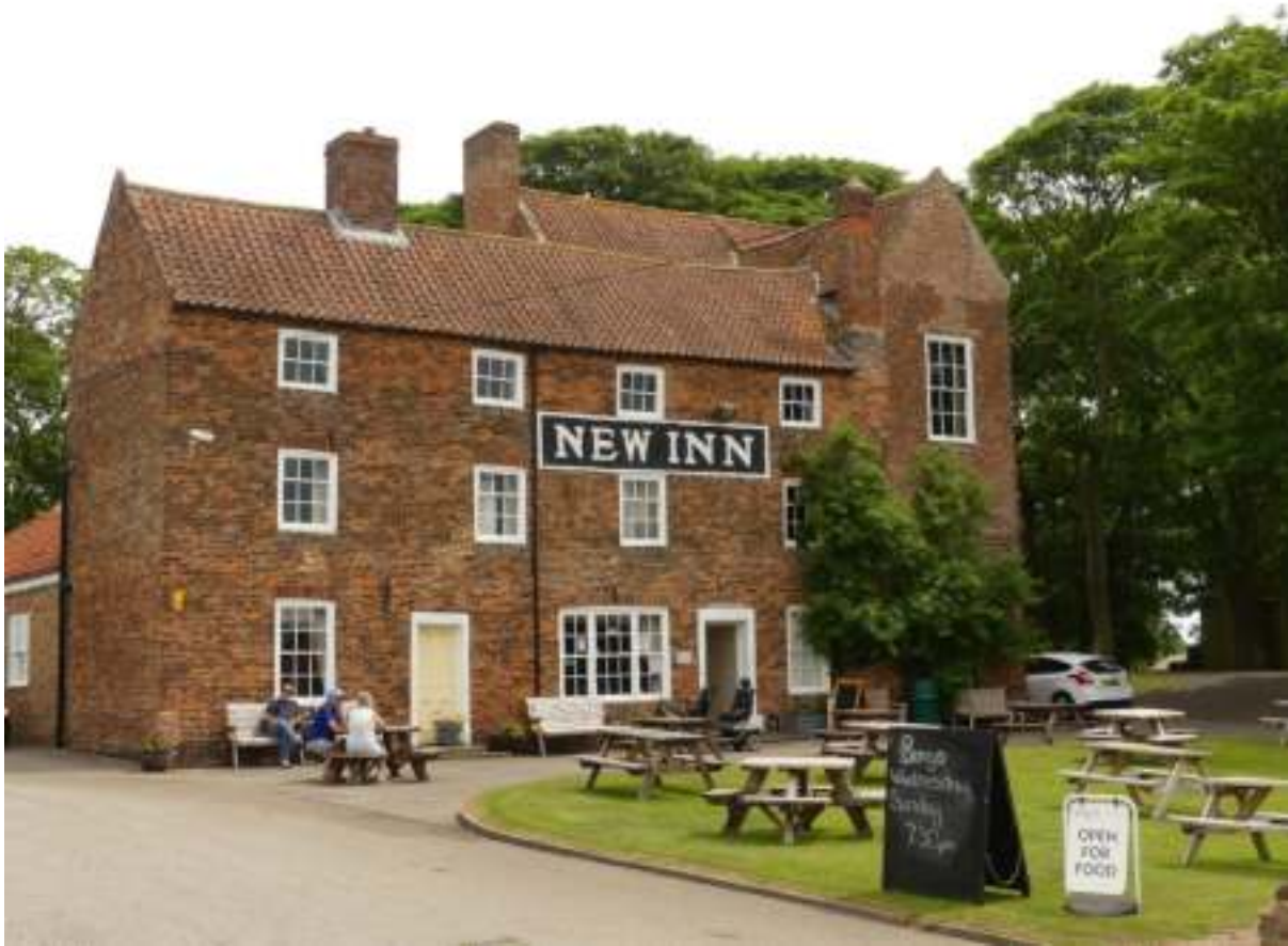
Figure 52: The New Inn at Saltfleet. This is a substantial seventeenth-century T-shaped building, the ‘Old Inn’, with a new additional north wing built in the later eighteenth century, leading to its renaming; it has been suggested that the original ‘Old Inn’ had its origins in the late sixteenth century.
